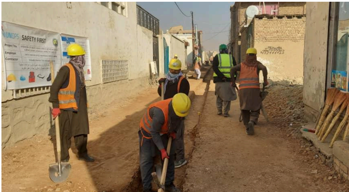
Photo 1: Drainage bed preparation in project Upgrading of Qala-e-Kaship streets with plum concrete surface (1080m), Gozar #14, District #5, Kabul City on 18 December 2023.
