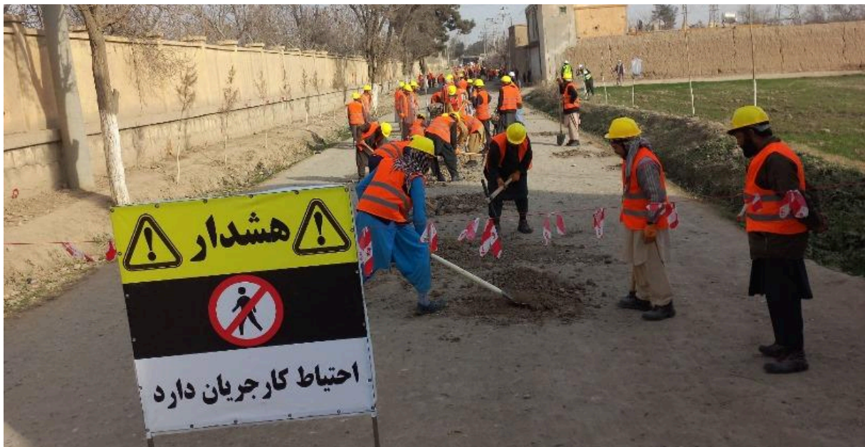
Photo 8: Subgraph preparation in project Construction of Naw Abad Sark#2 Karte-Zeraat Plum concrete surface Street from 0+000 to 0+ 700 in District-7 of Kunduz City on 21 December 2023.
