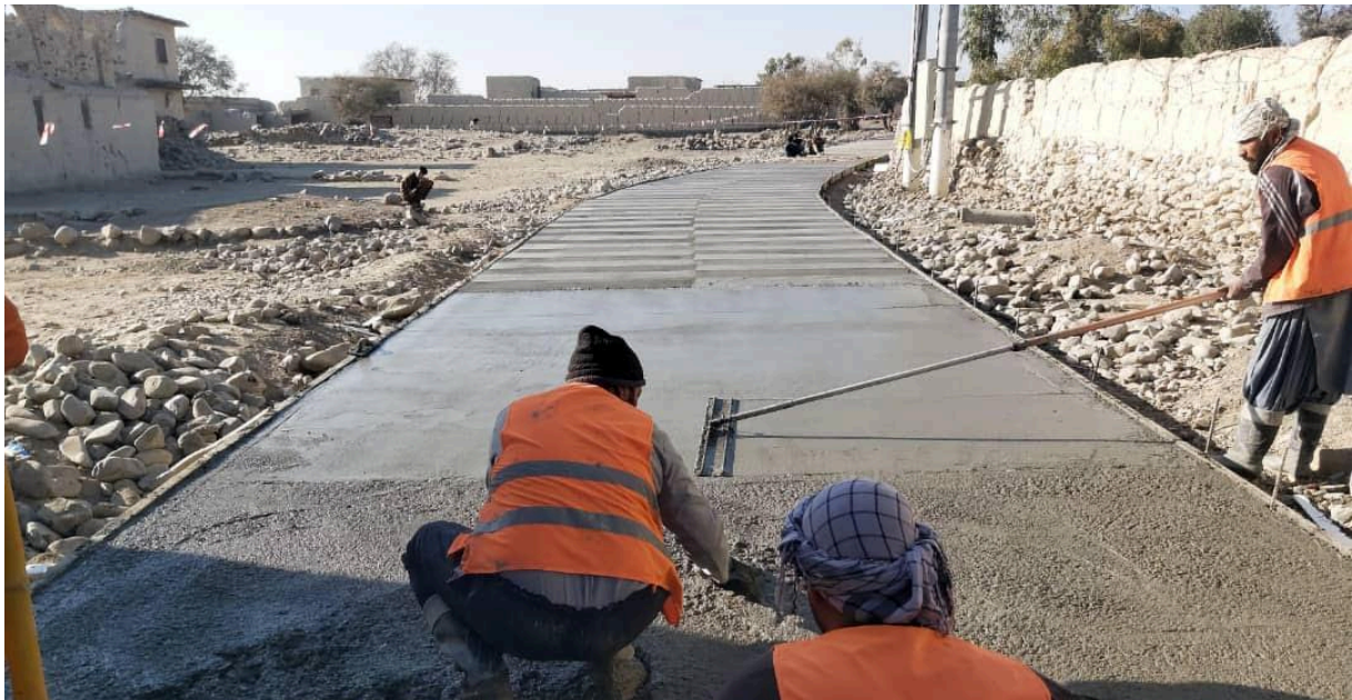
Photo 9: Street paving in project Upgrading of Khabash Khail Star-Kaly Road with the plum concrete surface (L-1380m) from (0+000 To 1+380) in Khost City on 26 December 2023.
